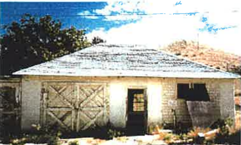
Garage and Metal Shop
