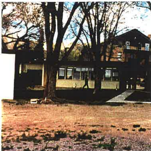
Class Room Annex
